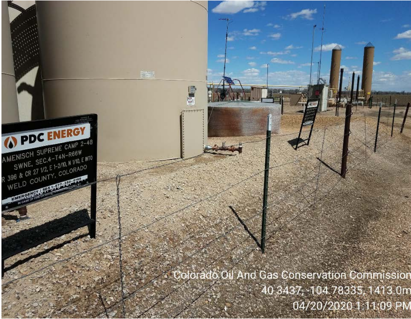
Earth berm on 4/20/2020
