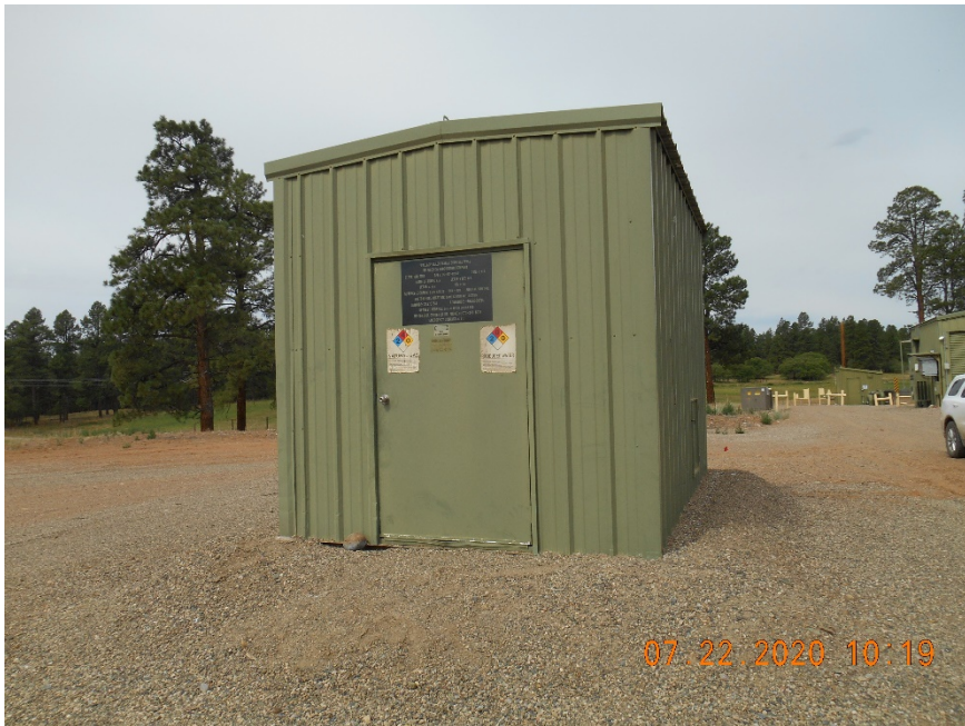
Injection wellhead housing with sign.
