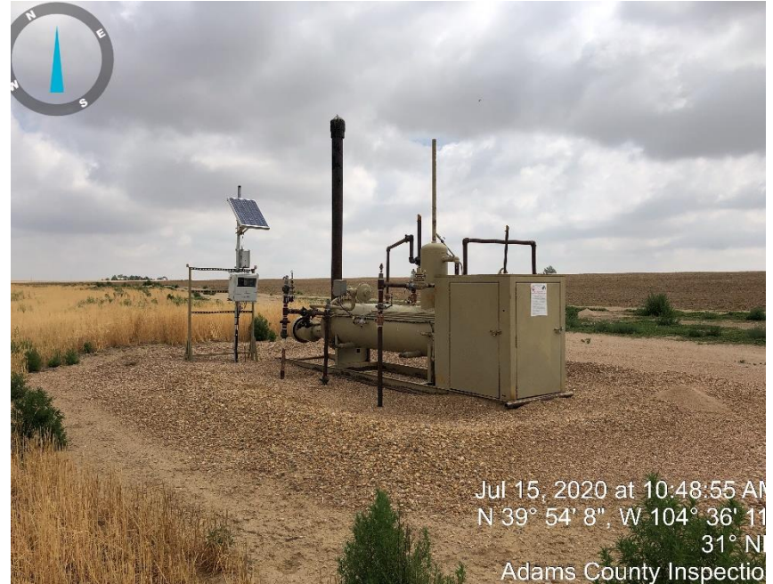
Photo #2 Meter and Separator.
