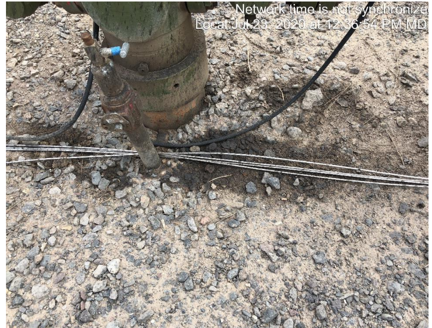
Photo #1598 Multiple places with stained soils by wellheads.
