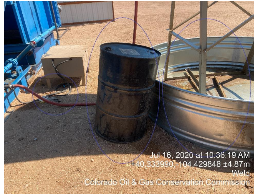
Photo #24 Trash, Barrel needs to be in secondary containment, Inadequate wildlife protections (netting) of secondary containments.
