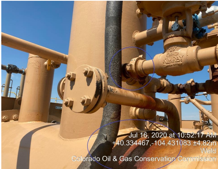
Photo #5 Appears to be leaking hammer unions at hi/low valves on various separators.
