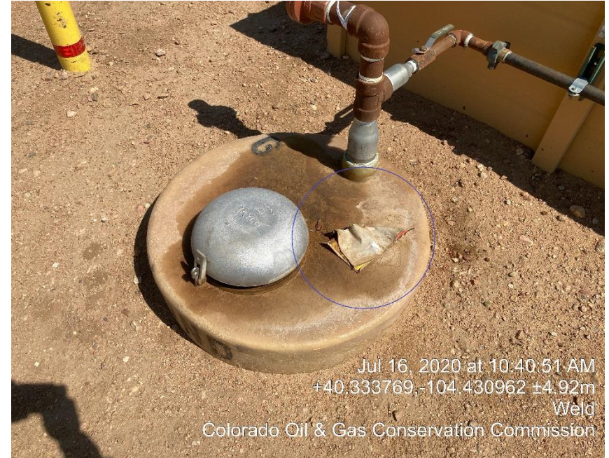
Photo #12 Unreadable placard/ missing capacity label
