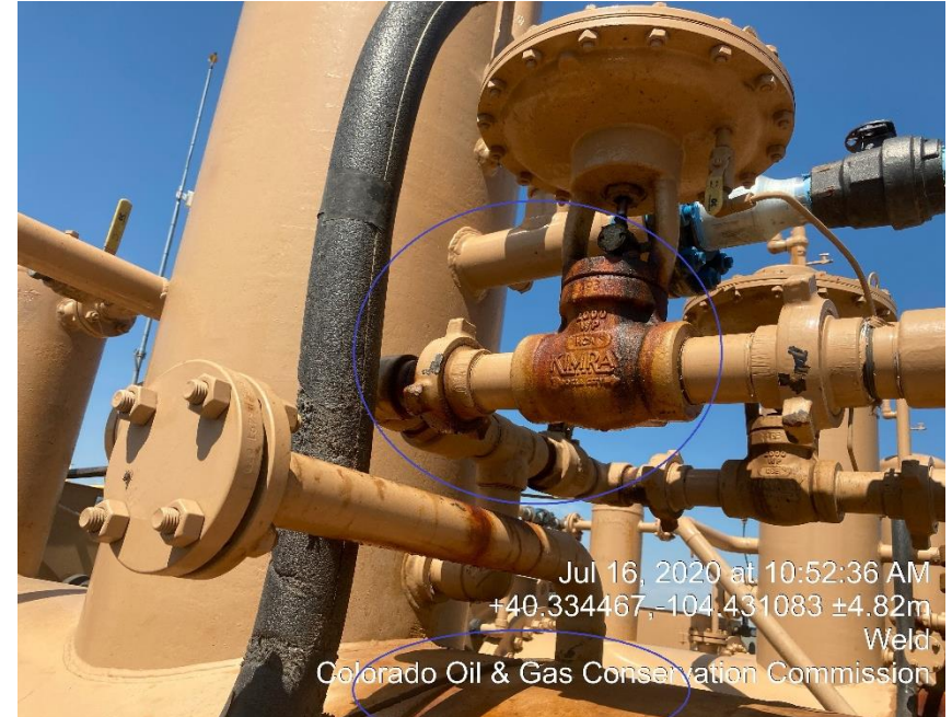
Photo #4 Appears to be leaking hammer unions at hi/low valves on various separators.
