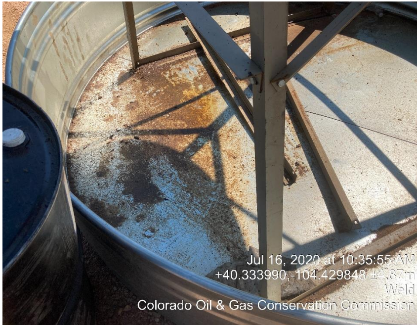
Photo #25 Inadequate wildlife protections (netting) of secondary containments.
