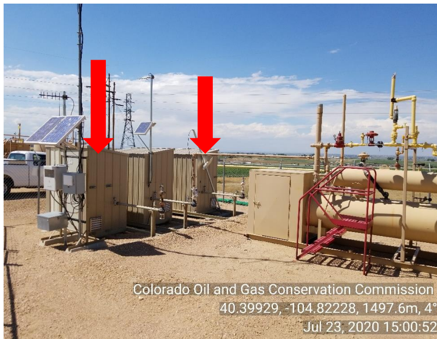
Photo 5: Unused/disconnected gas meters
