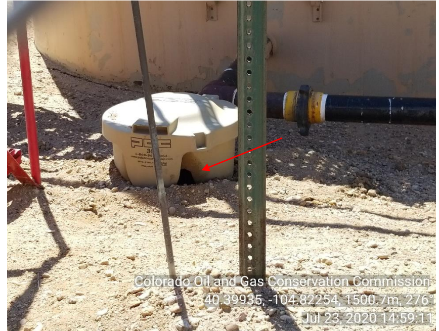
Photo 4: Hole in load out bucket
