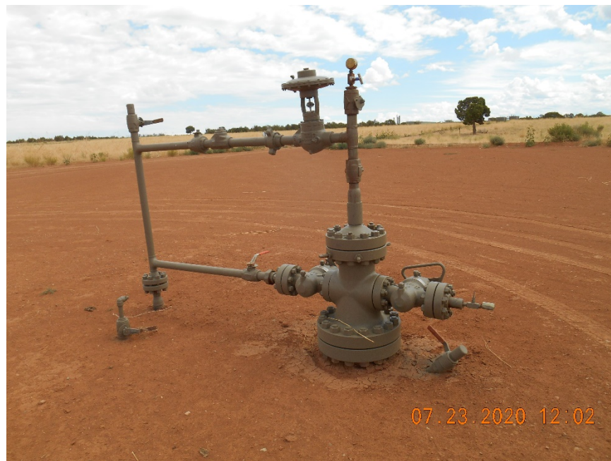
Injection wellhead.
