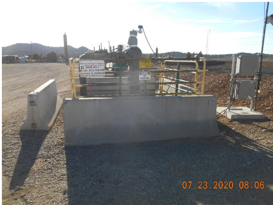
Injection wellhead with sign and fencing.
