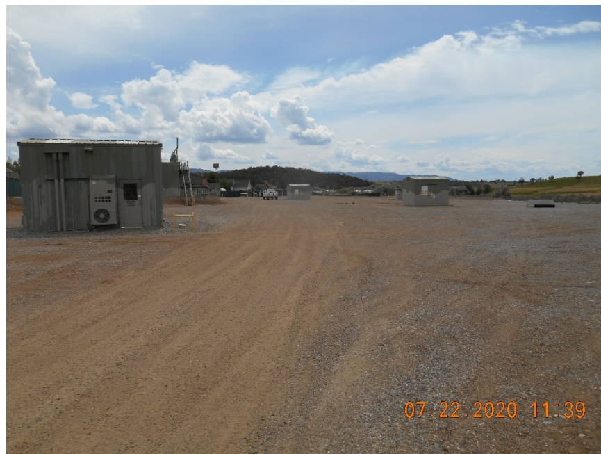
Location overview looking SE
