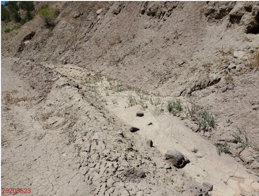
Photo 1: Photo taken from the west end of the Location, facing southwest. Photo shows areas of the stormwater diversion ditch where Halogeton was observed. Photo also shows sediment deposition within the ditch; Maintenance advised.
