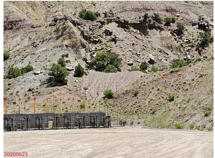
Photo 4: Photo taken from the Location facing northeast. Photo shows slopes on the northeast end of the Location with insufficient or missing BMPs to stabilize and protect slopes/soils.
