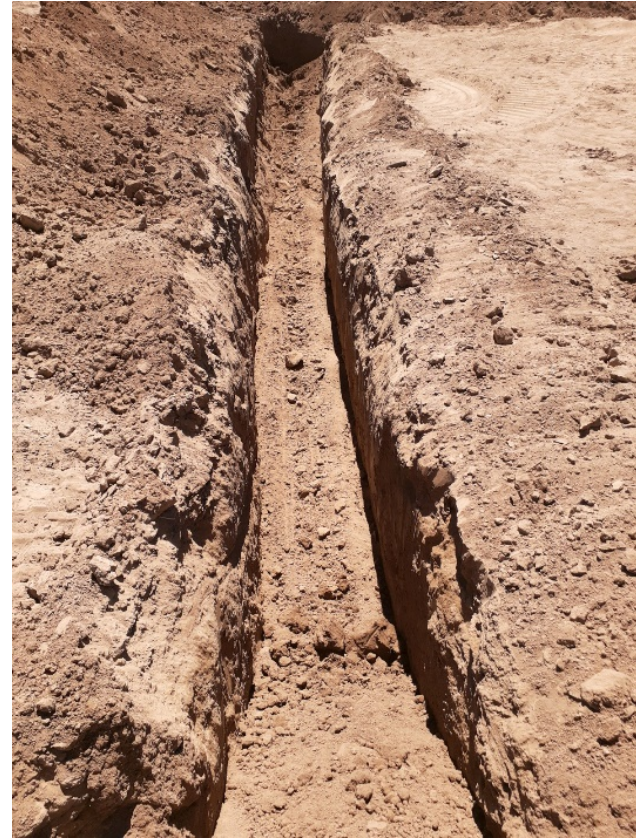
Flowline removed from excavation
