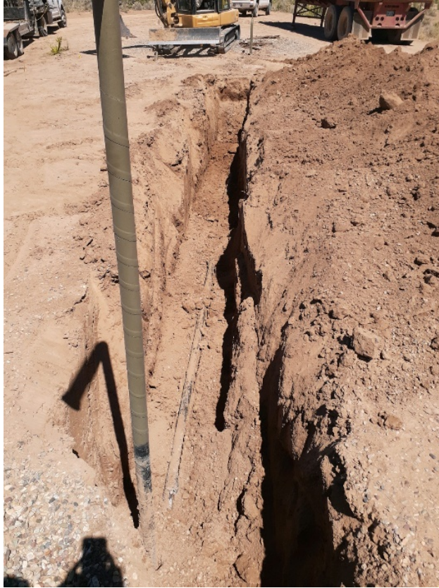
Flowline being exposed
