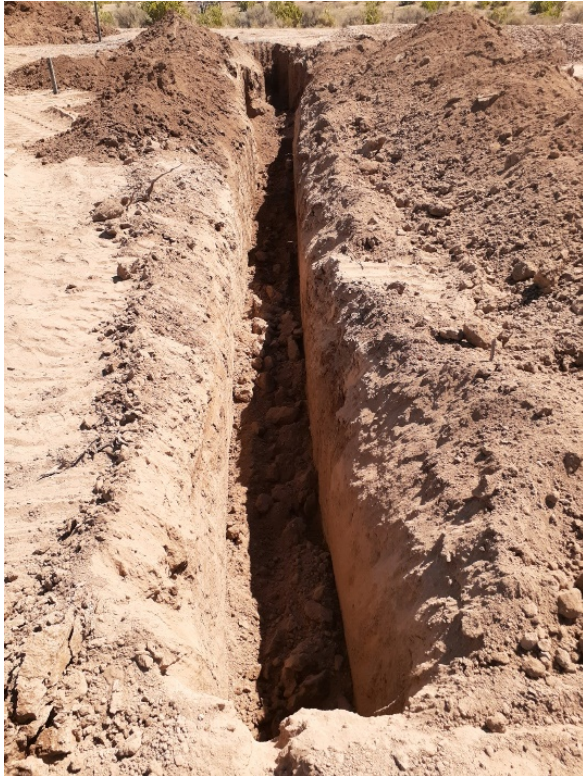
Flowline removed from excavation
