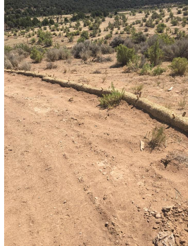
Stormwater BMP's installed
