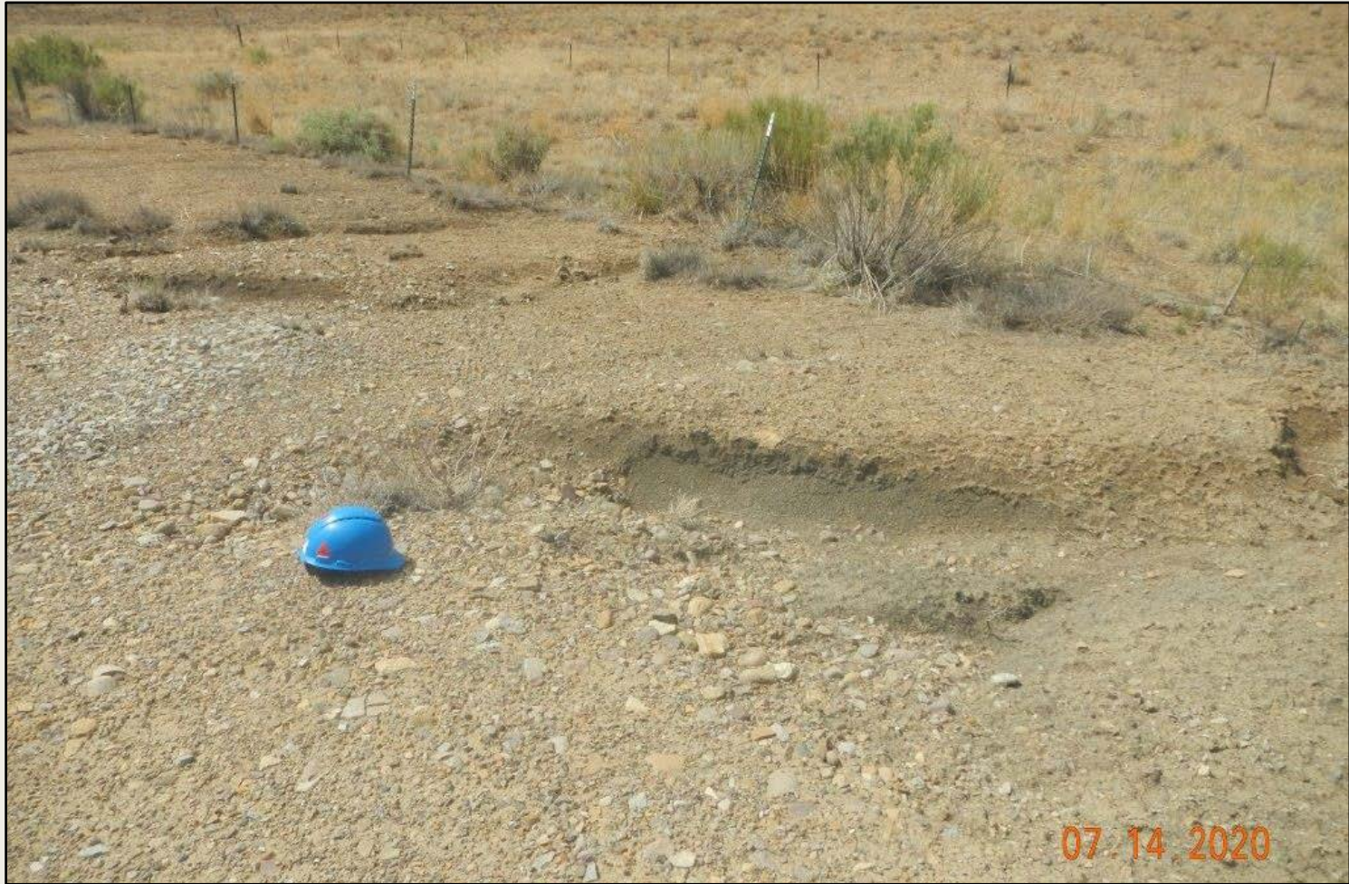
Photo 4. View of erosional channels flowing off of the southern portion of the well pad. Channels are approximately 1-2 feet deep and 2-4 feet wide and need stabilization.
