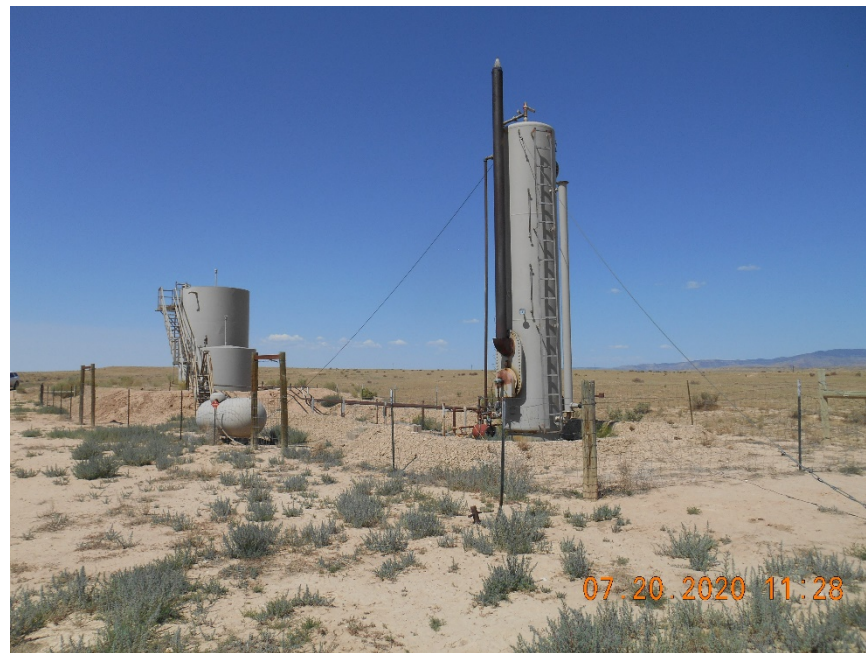
Vertical Separator with sign
