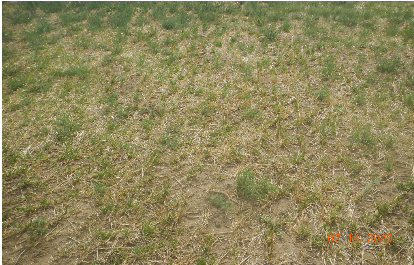
Photo 3. View of groundcover at the location shows soils were straw mulched for temporary stabilization. There is desirable grasses beginning to grow and also some undesirable weeds.
