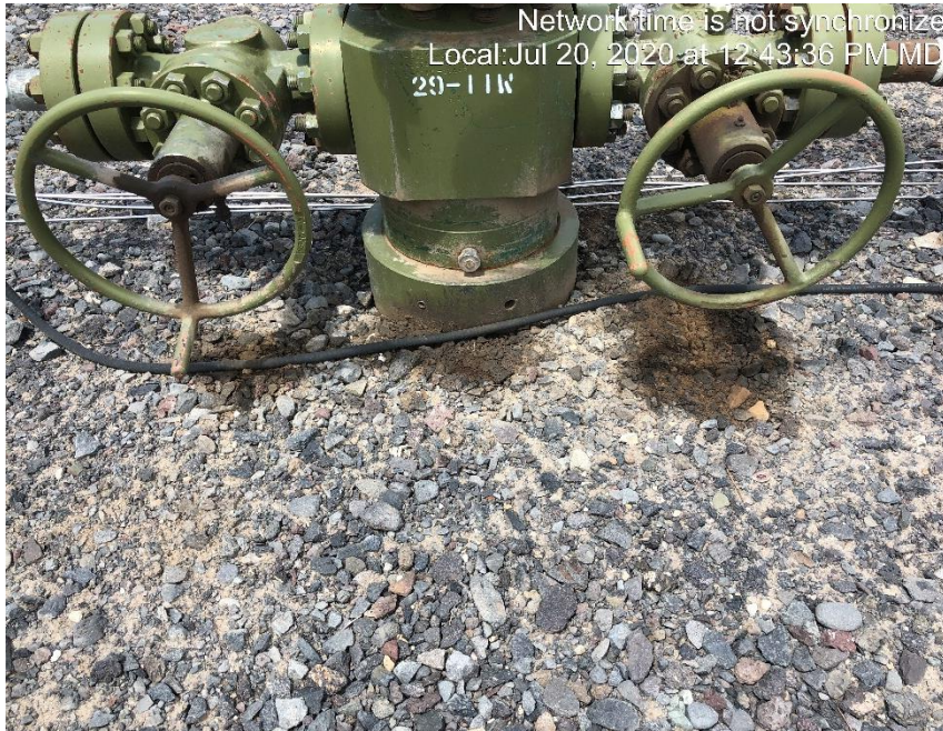
Photo #1562 Multiple places with stained soils at wellheads.
