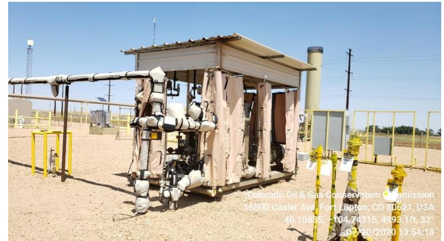
**Photo 11 Horizontal Heated Separators**
