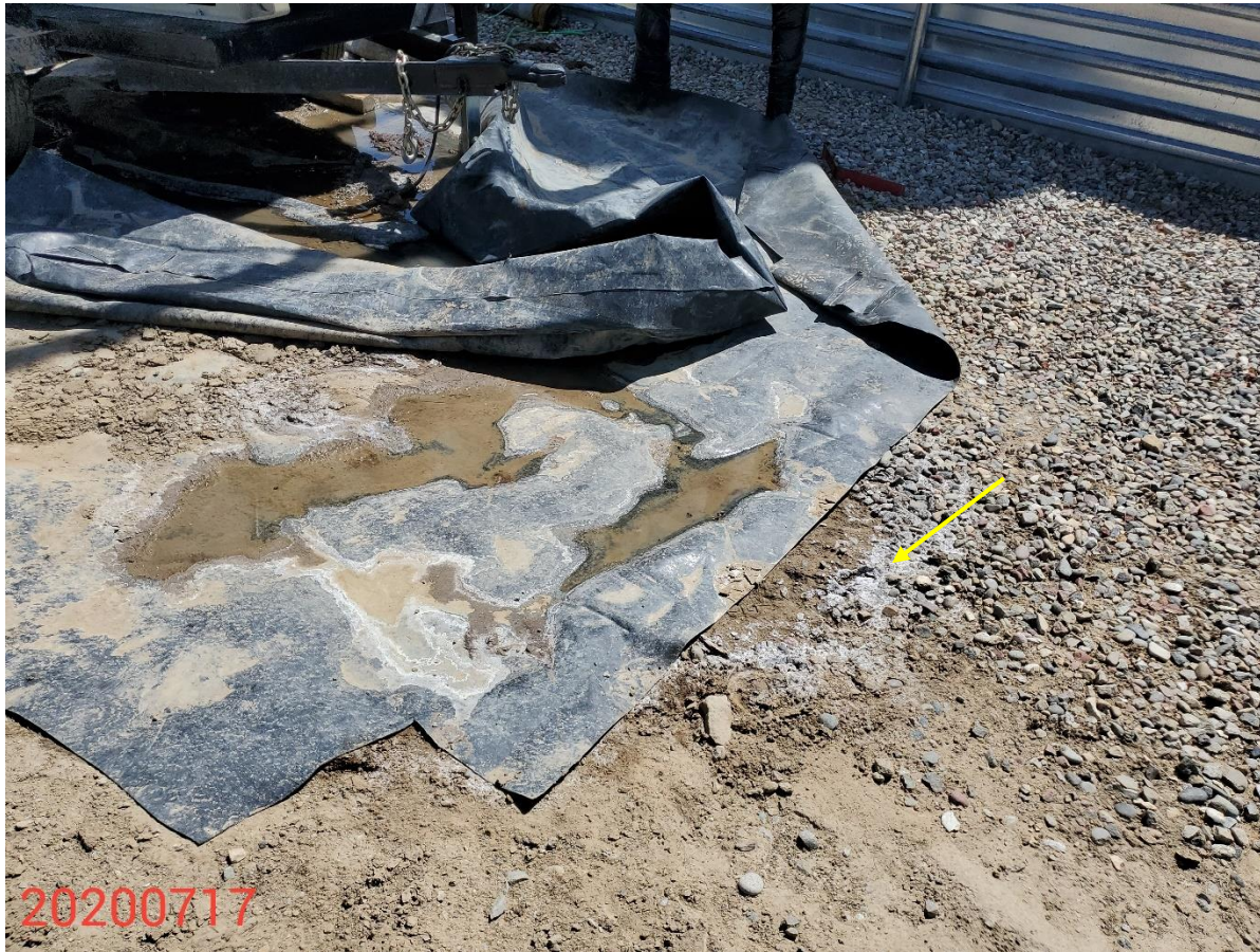
Photo 8: Continued from photo 7. Photo shows liner placed under the equipment is insufficient to contain spilled fluids and prevent discharge onto pad surface
