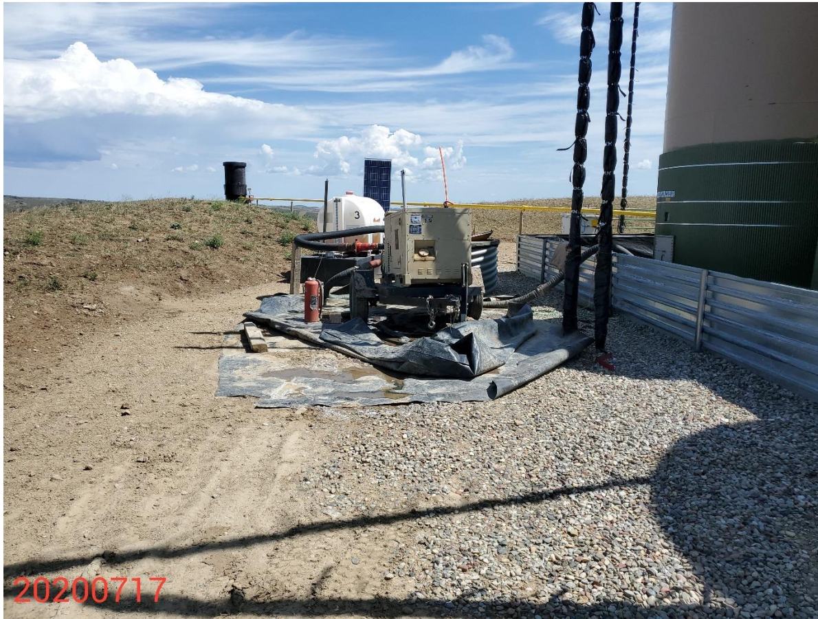
Photo 5: Photo taken from the northwest corner of the pad, facing north. Photo shows portable pumping unit; Small leak observed from a valve on the pump resulting in produced fluids discharging on to the pad surface.
