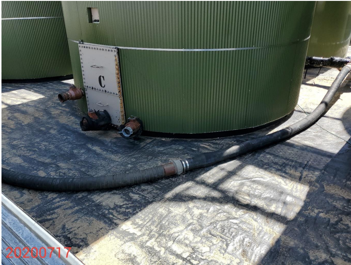
Photo 9: Photo taken west end of the tank battery. Photo shows pipe connecting battery to the pump.
