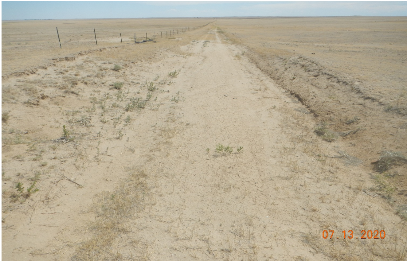
Photo 2. Facing south along portion of the access road which remains. This area of previous erosion has been regraded.
