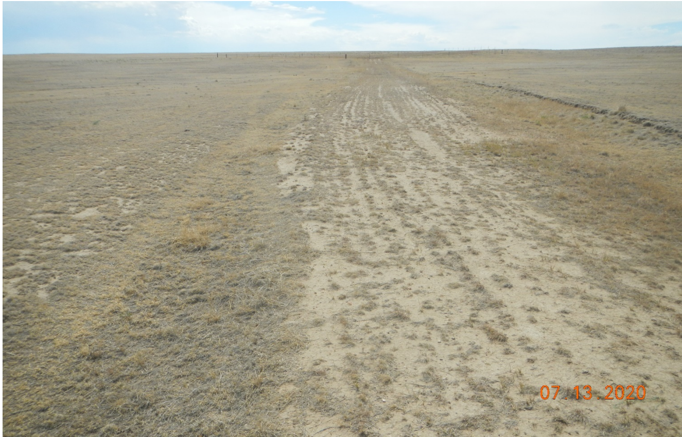
Photo 3. Facing west along the portion of the access road which has been reclaimed. This portion of the road has not reached 80% revegetation.
