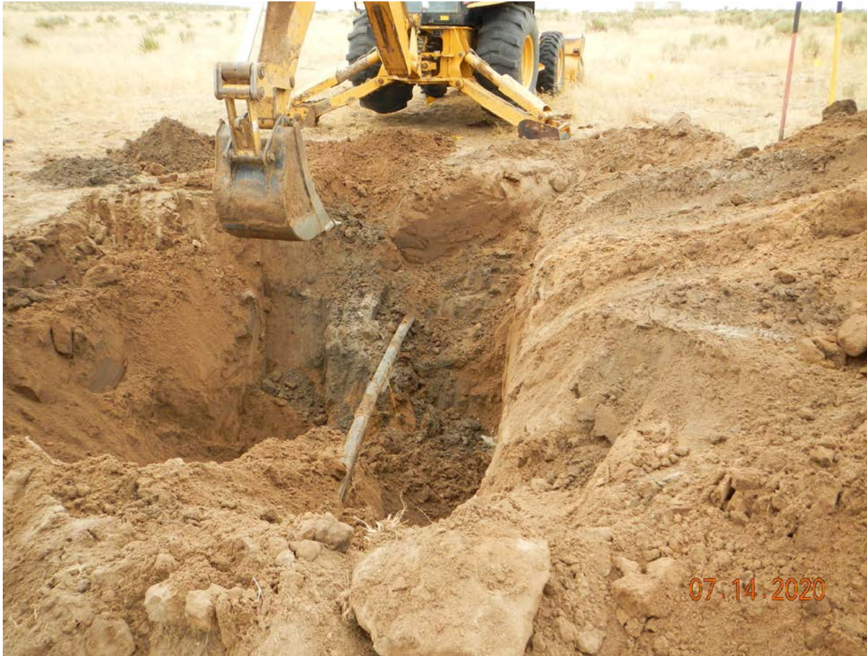
Photo # 10 – View east at flowline repair excavation. 2" poly water line, 3" poly gas line.
