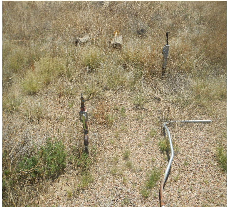
Photo 3. View of pipe risers with no LOTO.
