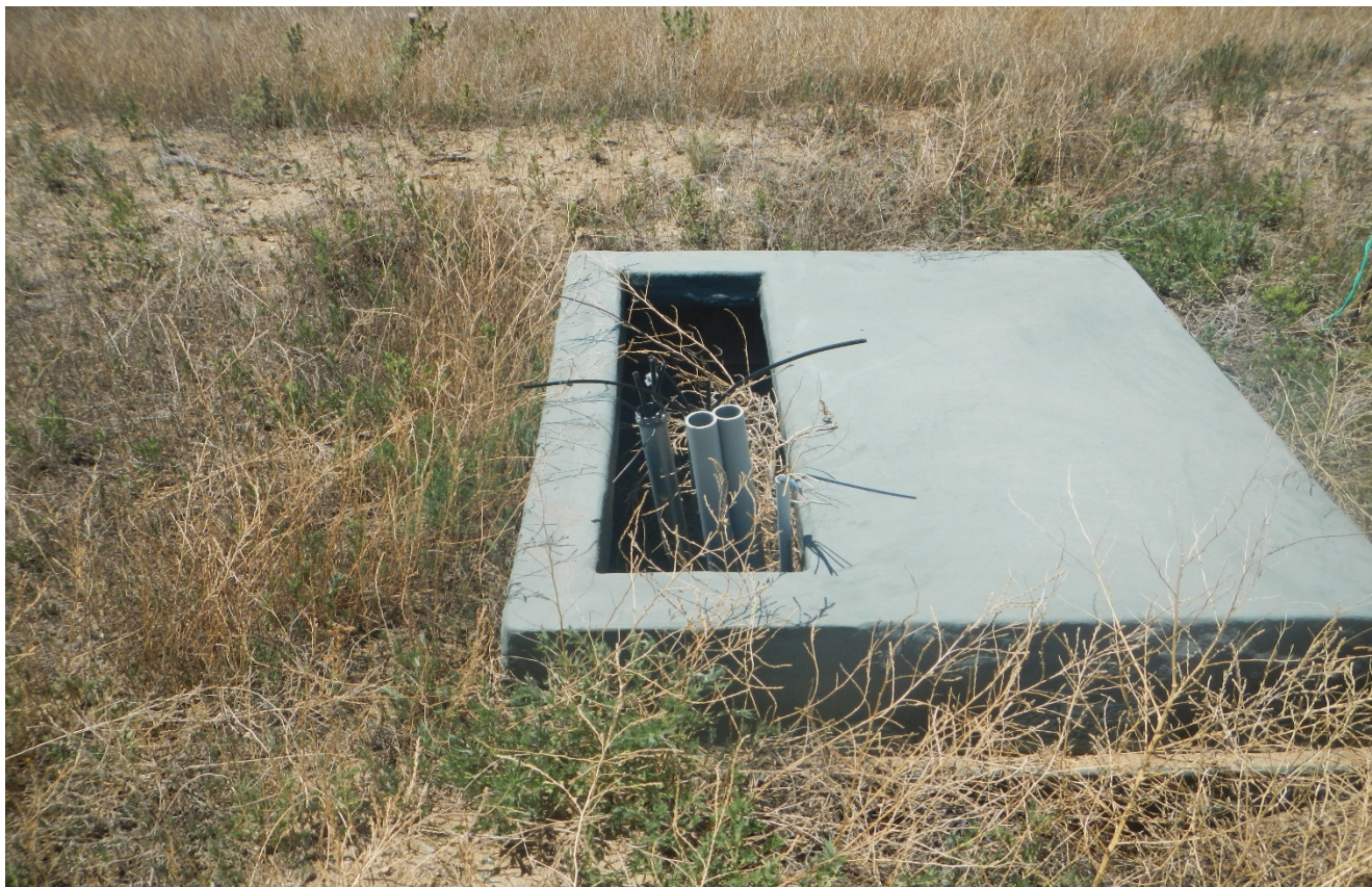
Photo 19. This cellar electrical box has exposed electrical wires.
