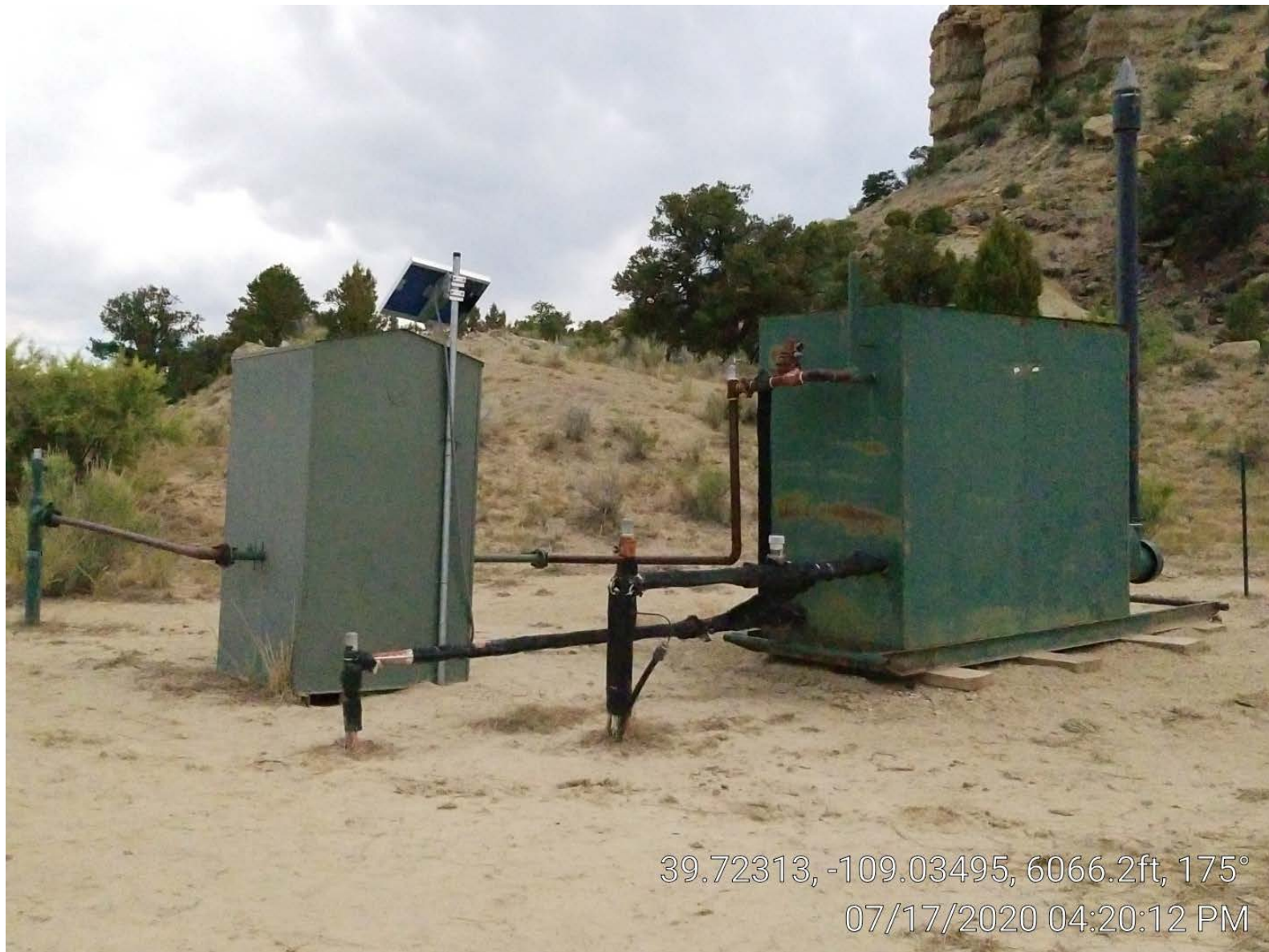
Photo 3. Meter building & separator.
