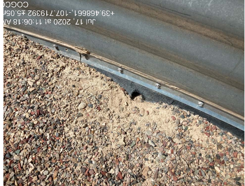
Multiple holes in tank battery containment bottom liner
