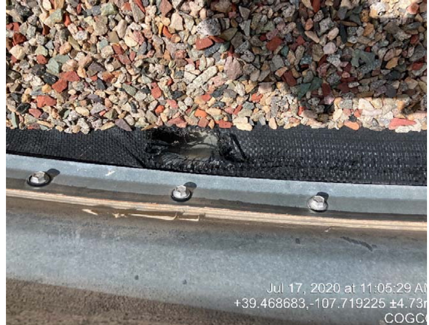
Multiple holes in tank battery containment bottom liner
