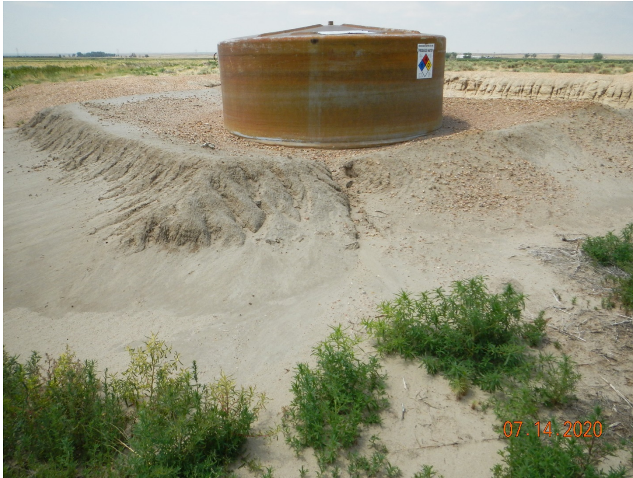
Photo # 11 – Berms need to be maintained north of skim tank
