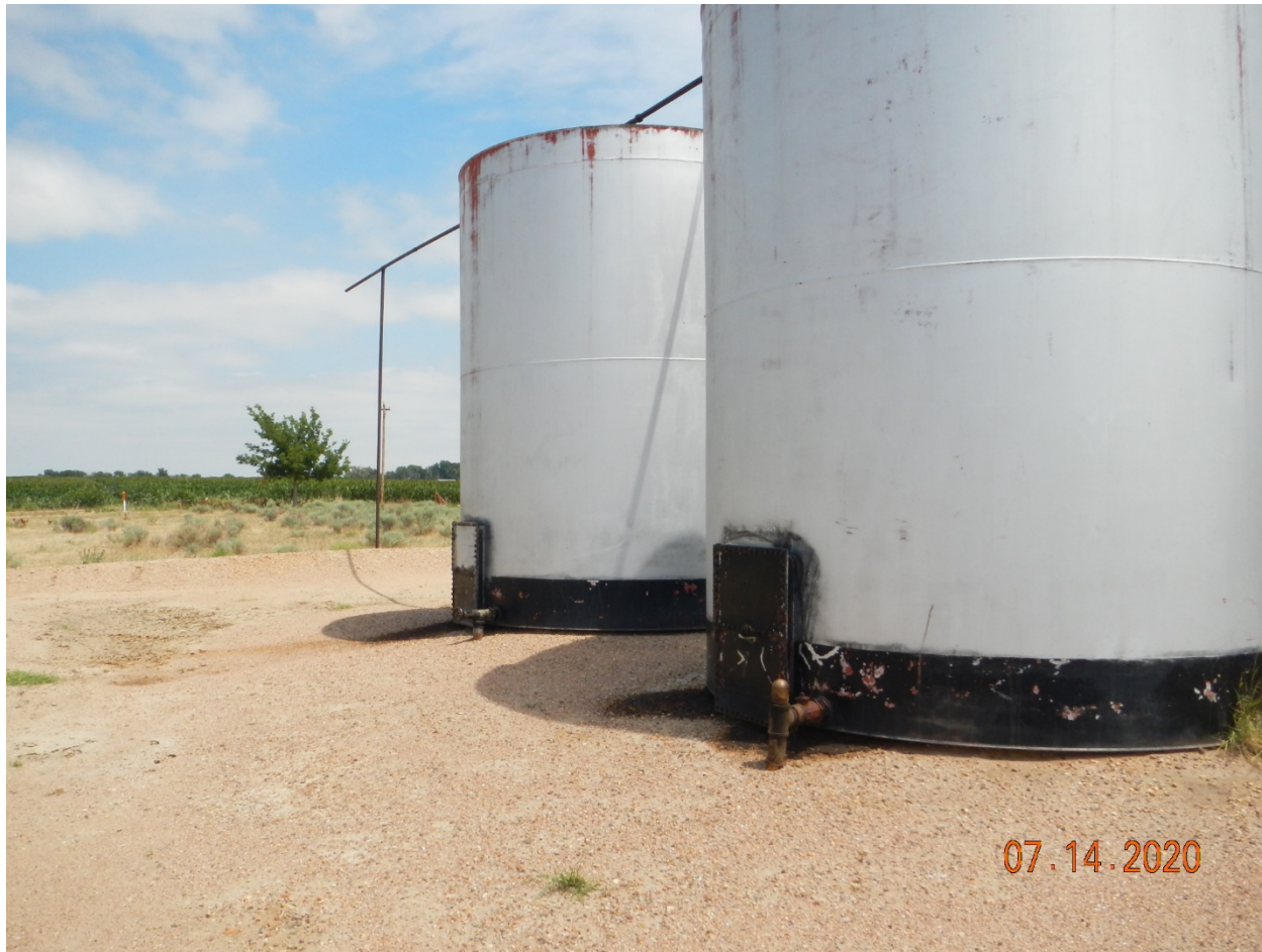
Photo # 2 – West side of tank battery, oily soil under tanks and valves
