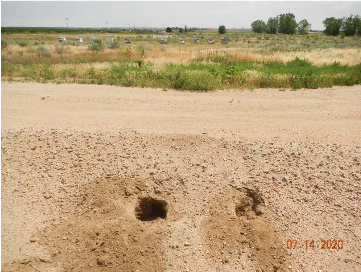
Photo # 4 – East side berm of tank battery, animal burrows
