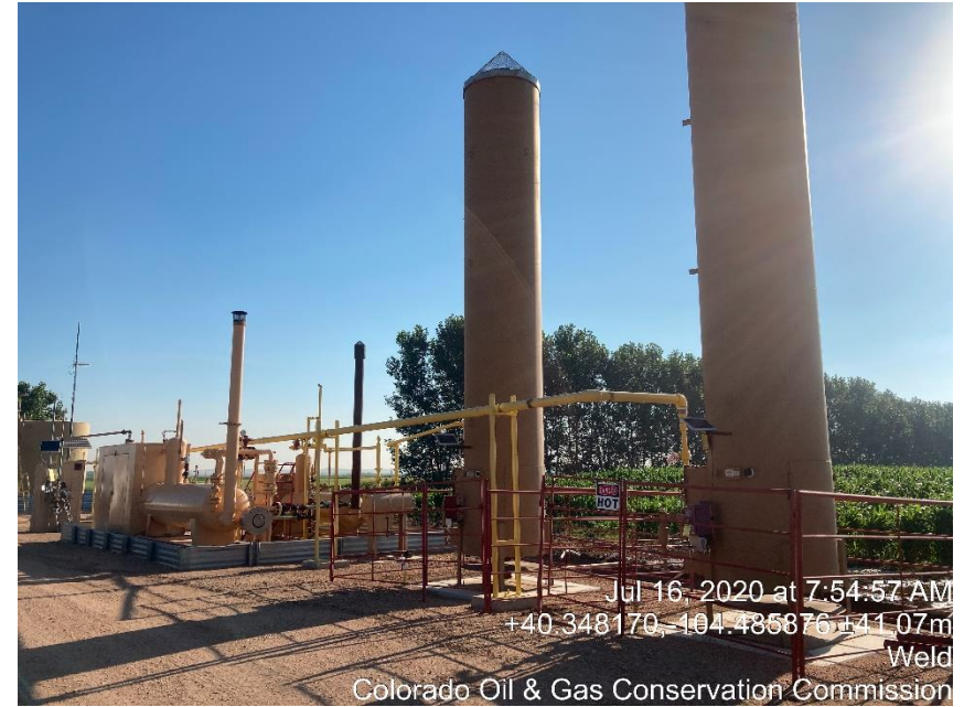
Photo #2 Separators, ECD's & Meter Run
