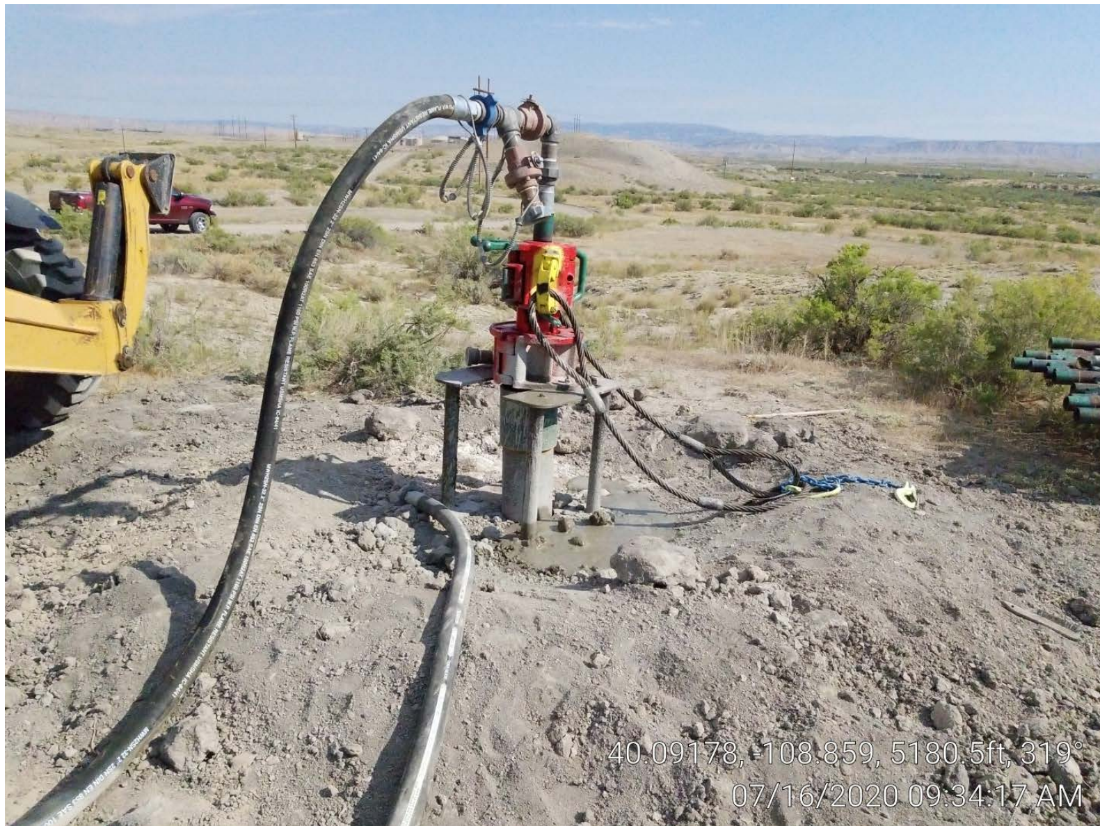
Photo 1. Cement pumped into well.
