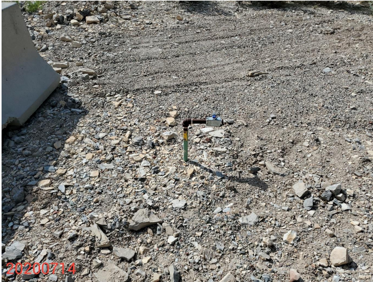
Photo 12: Photo of riser on the west end of the Location.
