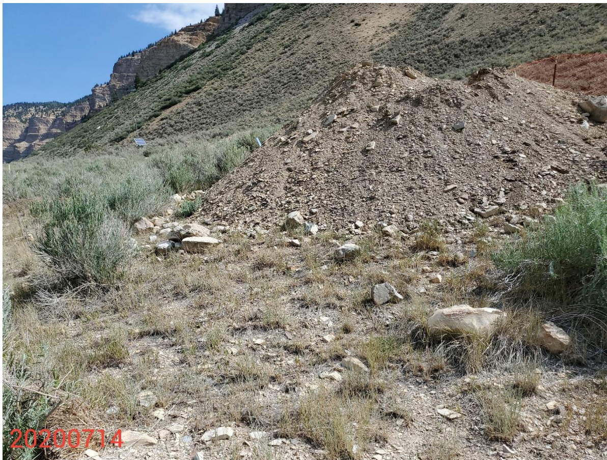
Photo 3: Photo taken from the west end of the Location, facing northeast. Photo shows BMPs to prevent sediment transport from the soil stockpiles are missing or insufficient.
