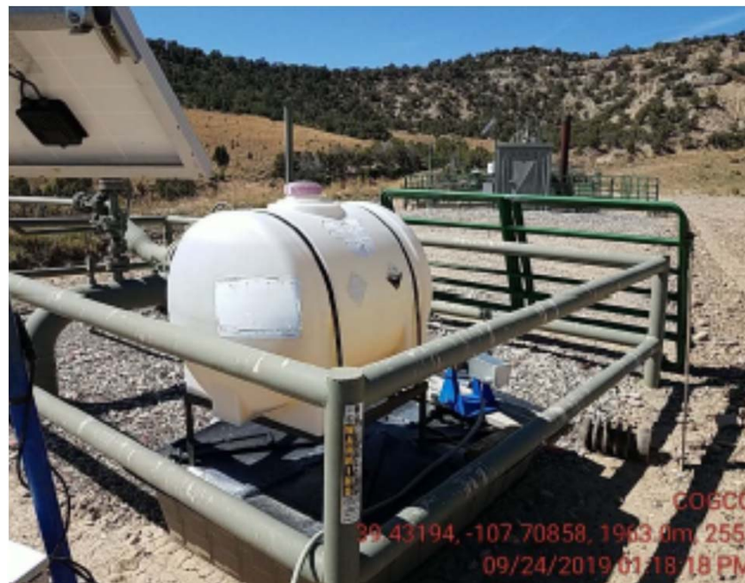
previous inspection photo of chemical tank
