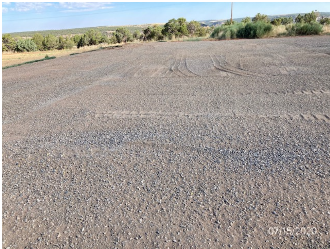
YF-3 Well Location: Area where impacted soil was has been backfilled with clean \frac{3}{4} inch road base.
