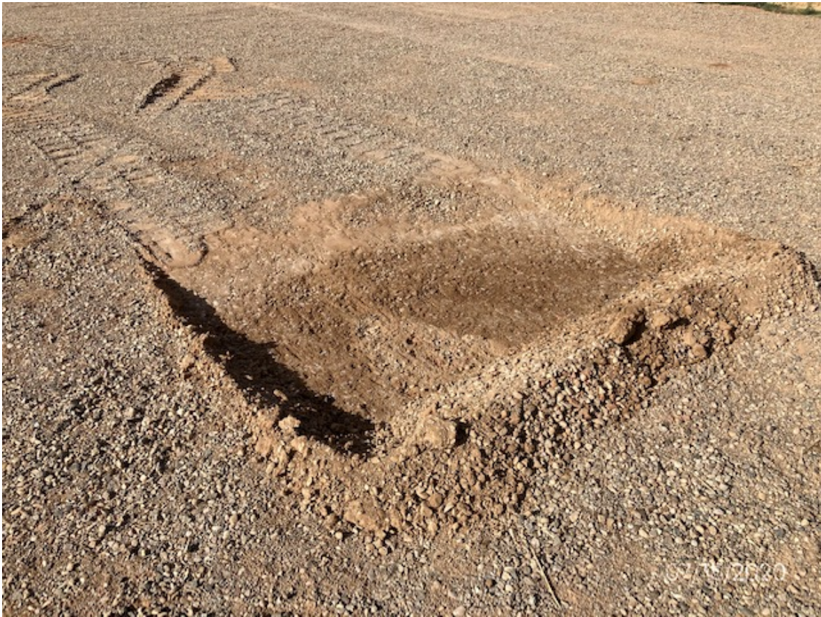
YF-3 Well Location: Impacted soil being removed from current location.
