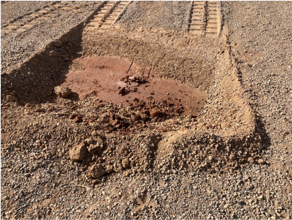
YF-3 Well Location: All impacted soil has been removed from YF-3 Well Location.
