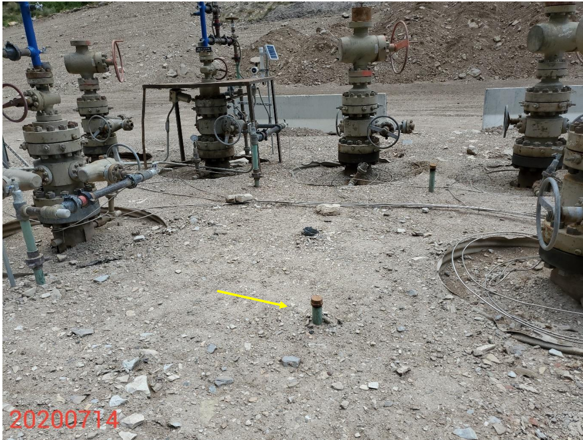
Photo 1: Photo taken from the PA well GPS position. Photo shows riser remaining.
