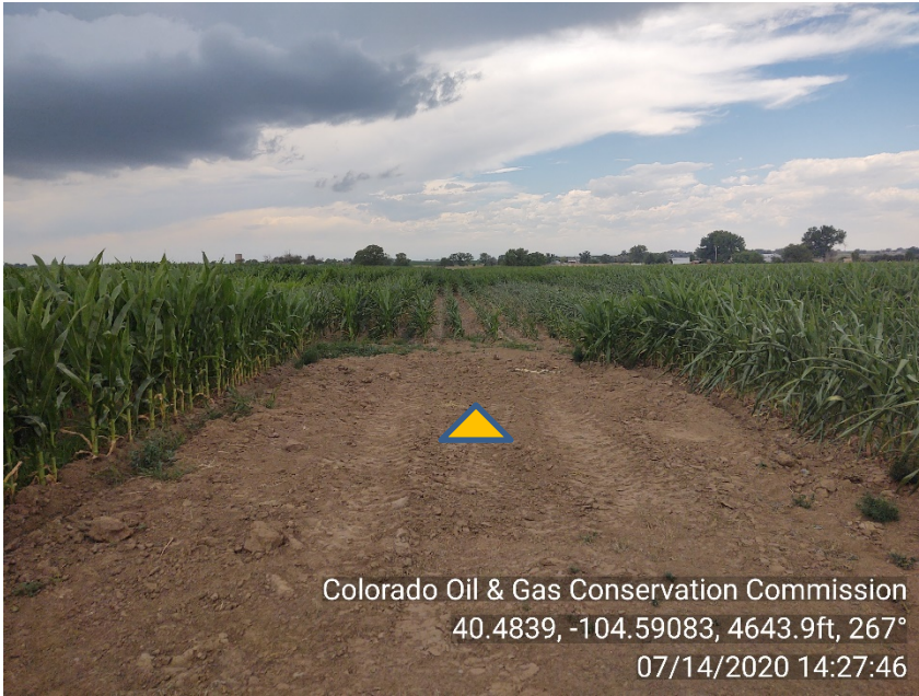
Photo #1 Foose A18-10 (05-123-13855) Wellsite Plugged & Abandoned | PA ~ 5 yds. Reclamation progressing
