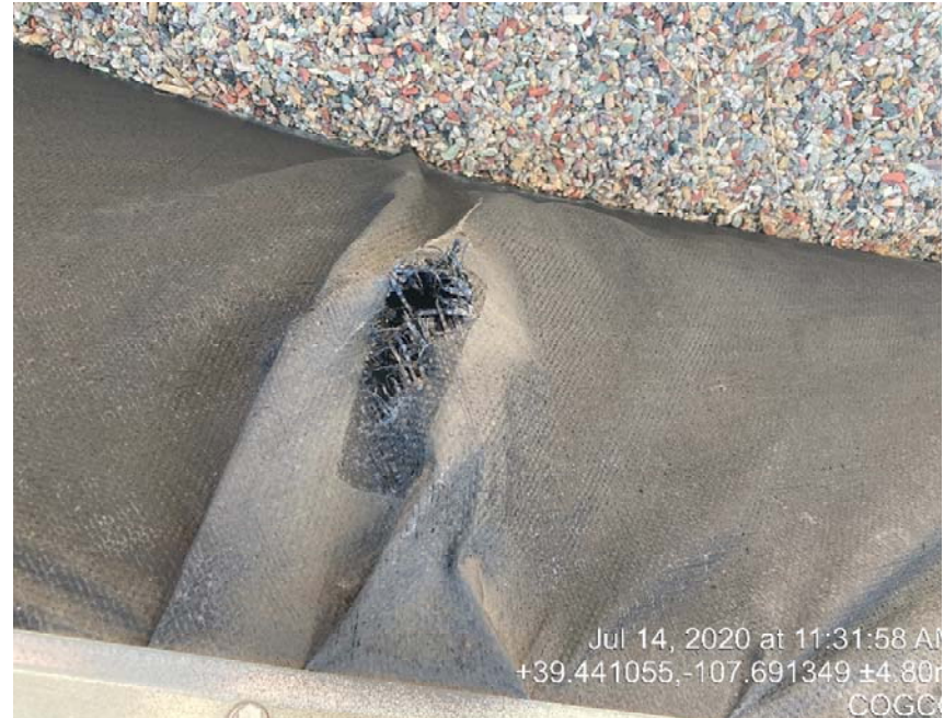
Holes in containment
