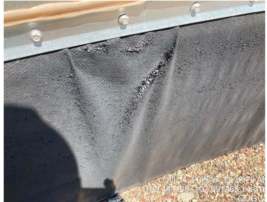
Holes in containment
