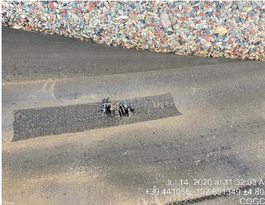
Holes in containment
