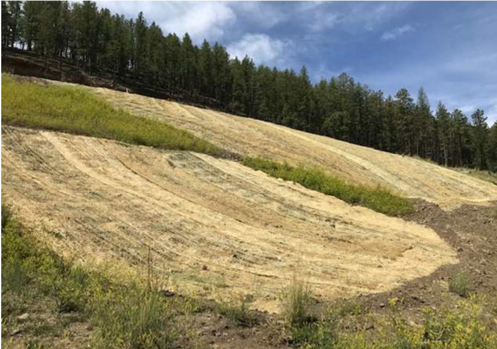
PHOTO 2: THE FILL SLOPE WAS RECONTOURED TO MATCH THE SURROUNDING SLOPE. THE DISTURBANCE WAS SEEDED WITH AN APPROVED CPW SEED MIX AND EROSION CONTROL BLANKETS WERE INSTALLED OVER DISTURBED AREAS. THE EXISTING DIRT BERM AT THE TOE OF THE SLOPE AND EXISTING VEGETATION WILL PROVIDE SEDIMENT CONTROL.
