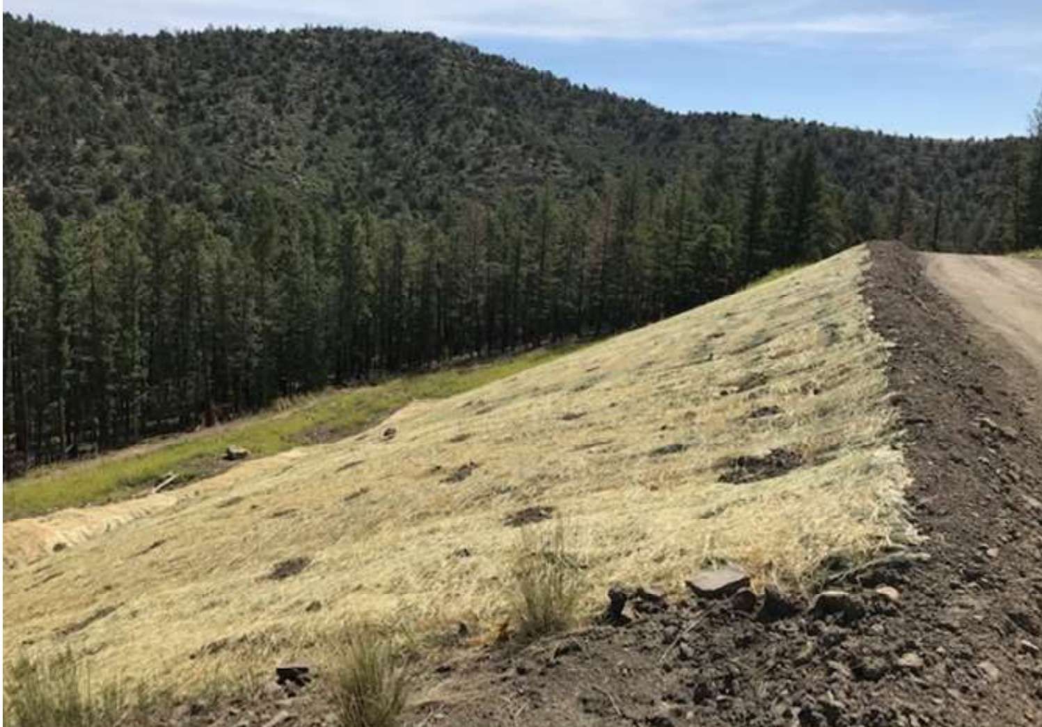
PHOTO 1: THE FILL SLOPE WAS RECONTOURED TO MATCH THE SURROUNDING SLOPE. THE DISTURBANCE WAS SEEDED WITH AN APPROVED CPW SEED MIX AND EROSION CONTROL BLANKETS WERE INSTALLED OVER DISTURBED AREAS. THE EXISTING DIRT BERM WILL PROVIDE ADDITIONAL EROSION CONTROL.
