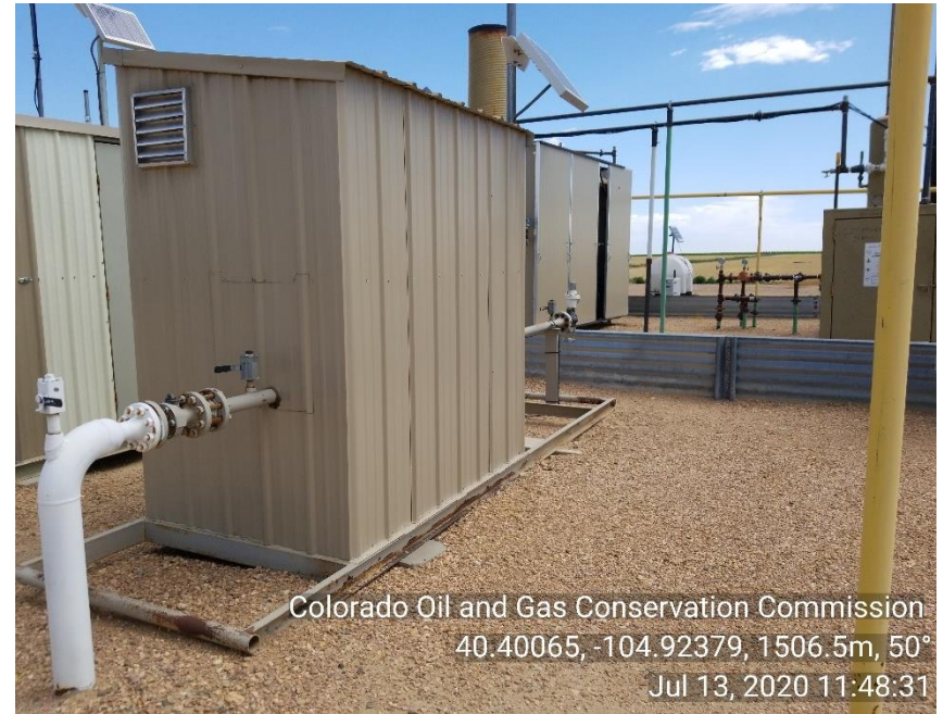
Photo 6: Unused/disconnected gas meter
