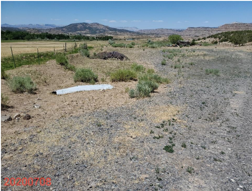
Photo 1: Photo taken from the south end of the Location, facing Northwest. Photo shows Location has not been reclaimed; Various pipe and debris appears to be stored on the Location. Gravel has not been removed; Compaction alleviation, recontouring/regrading and revegetation activities have not been conducted.
