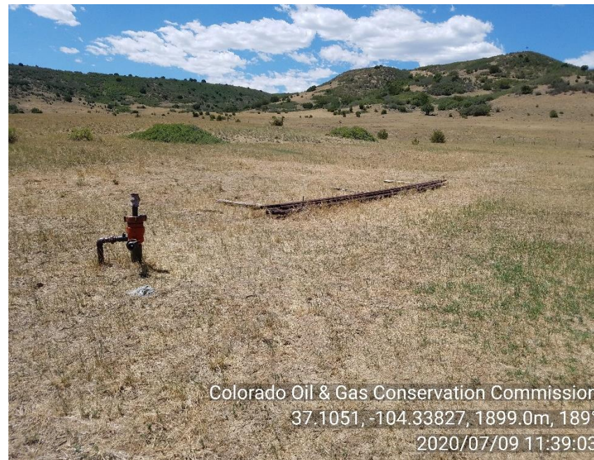
PHOTO 2: UNUSED EQUIPMENT STORED ON LOCATION (SEVERAL JTS OF TBG). REMOVE UNUSED EQUIPMENT PER RULE 603.f. CA DATE 10-9-2020
