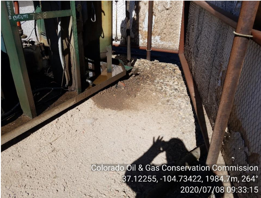
PHOTO 3: AREA OF IMPACTED SOIL NEAR LOW CORNER OF COMPRESSOR SKID. Conduct maintenance on equipment, cleanup stained material and review self inspection processes PER RULE 1002.f.(2)F. CA DATE 7-20-20.
