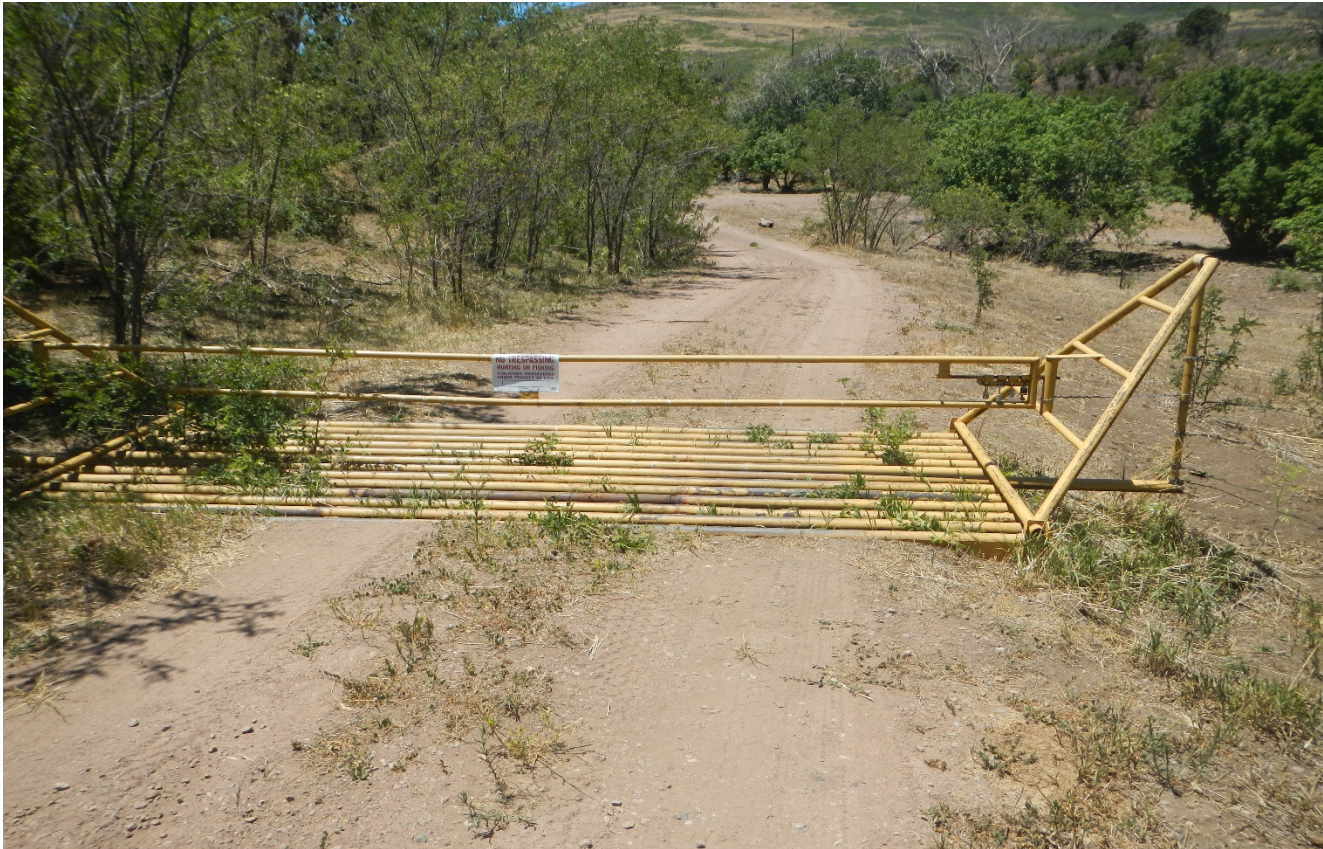
Photo 1. Facing west at the beginning of the access road. The access road has not been reclaimed and the cattle guard and gate remain.
