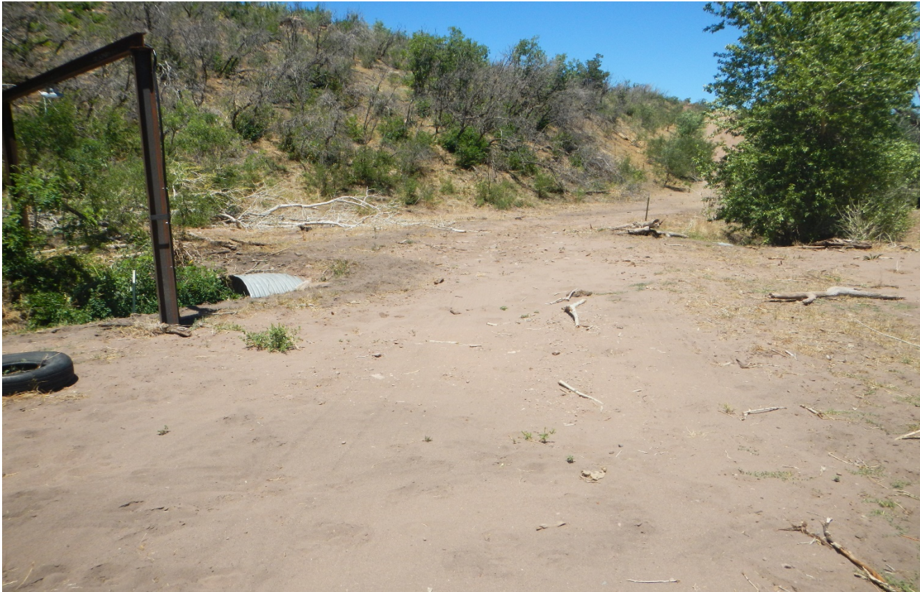
Photo 2. Facing northeast where road crosses the stream. Road was not reclaimed and culvert remains.
