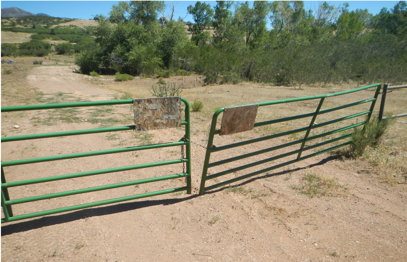
Photo 1. The gate at the beginning of the access road has fallen off the hinges and needs to be repaired.
