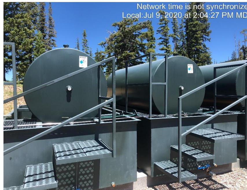
Photo #1498 Multiple tanks missing required information.
