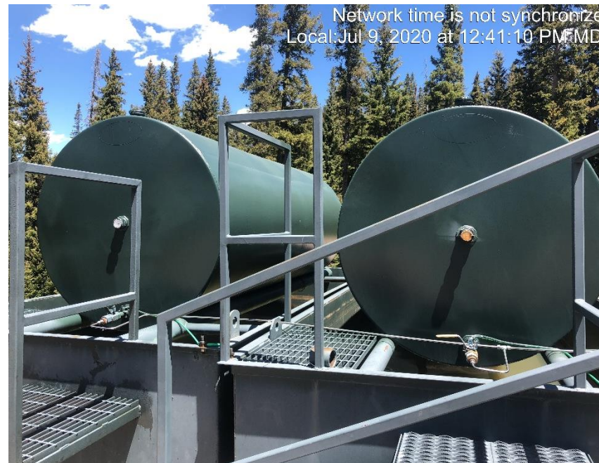
Photo #1491 Multiple tanks missing required information.
