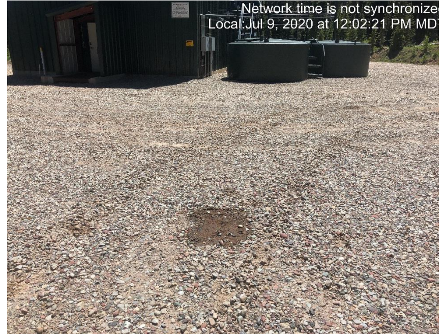
Photo #1489 Multiple places with stained soils outside of containment.
