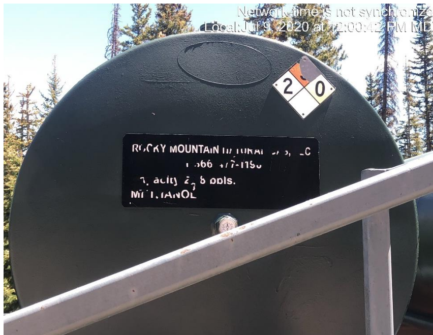
Photo #1486 Tank label weathered and not legible.
