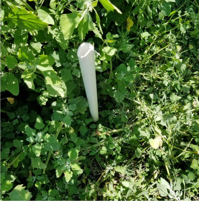
Photo 3 – Broken monitoring well
