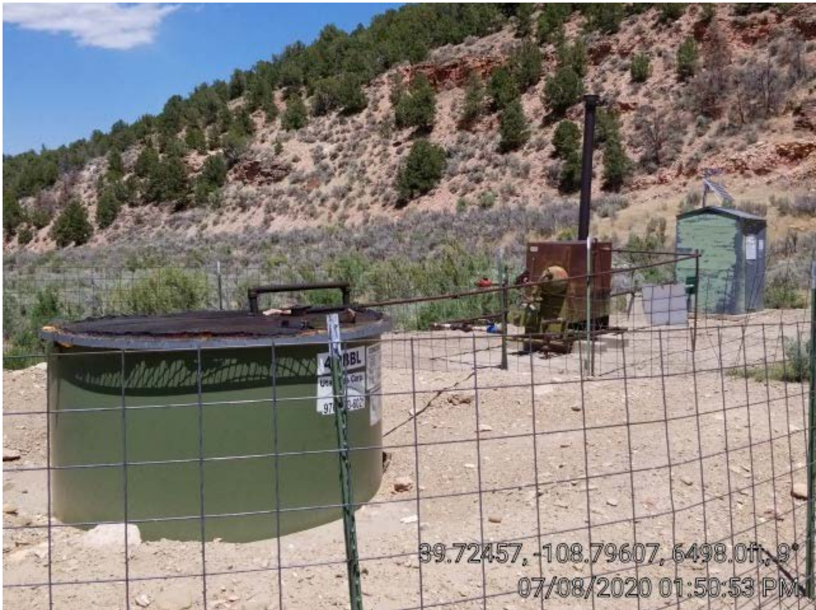
Photo 2. Tank, separator, and meter building.
