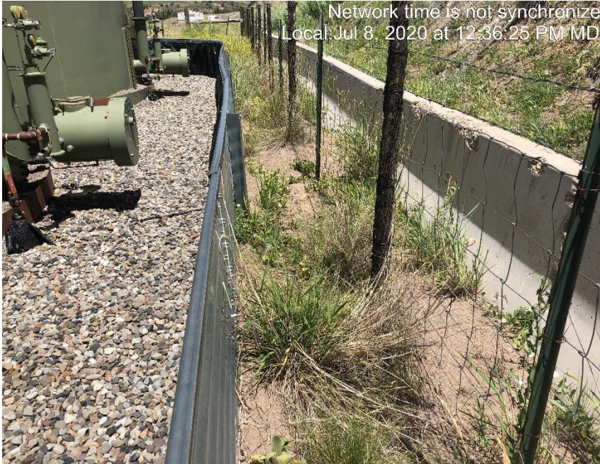
Photo #1478 Weeds encroaching on tank containment.
