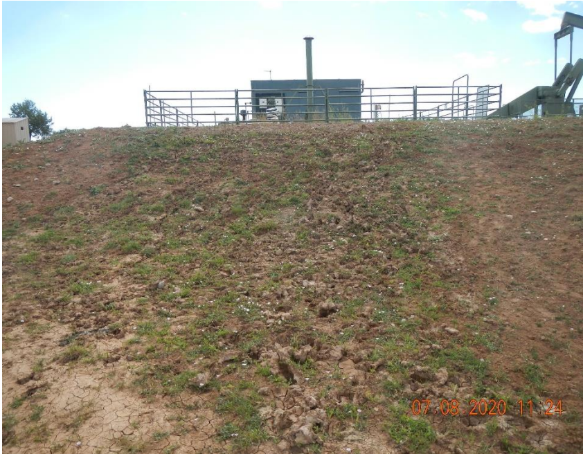
Flow path of produced water to the west, off of location. Evidence of flow and staining present for ~300'.
