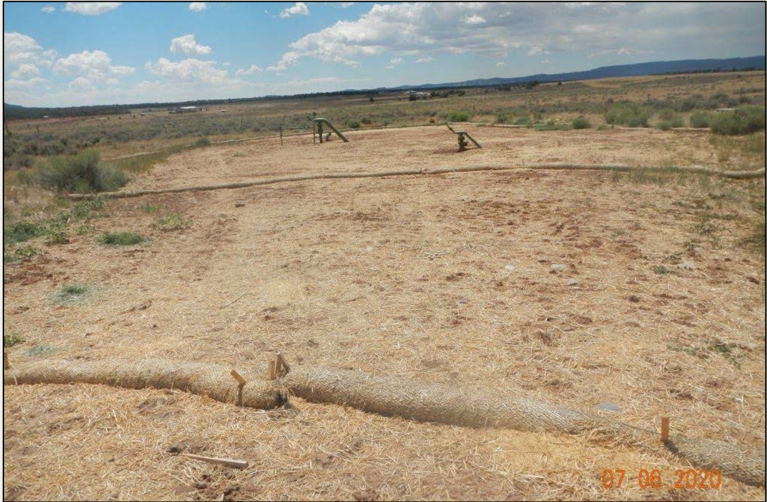
Photo 1. View of the western project area from the center of the well pad facing westward. Wattles are trenching and staked in place, and appear to be functioning.
