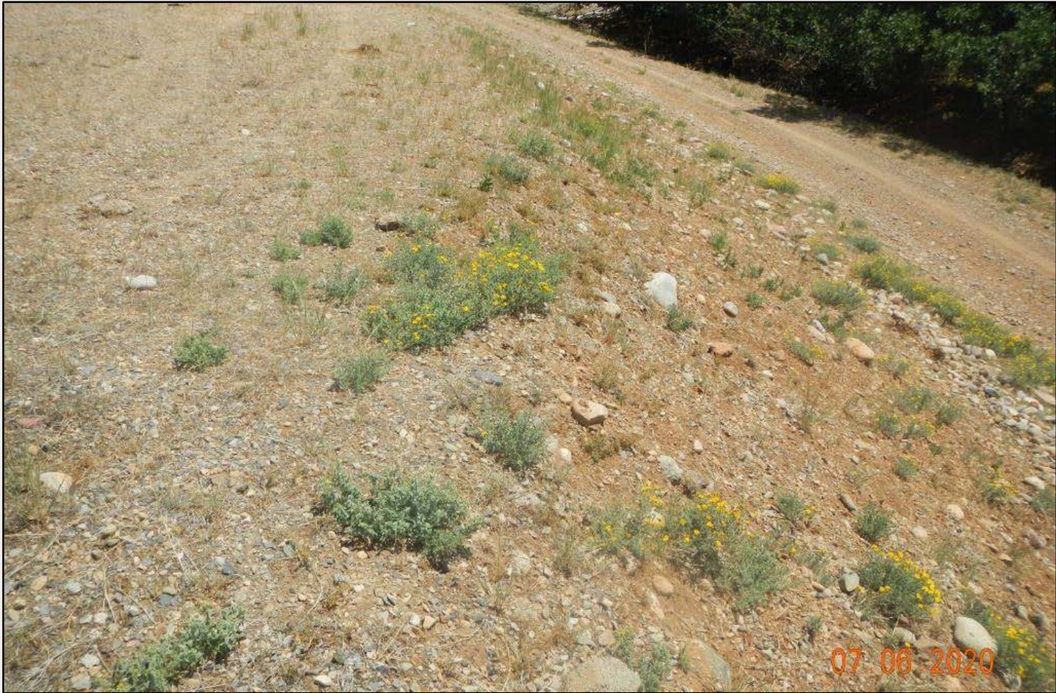
Photo 3. View of the southwestern fill slope facing eastward.
