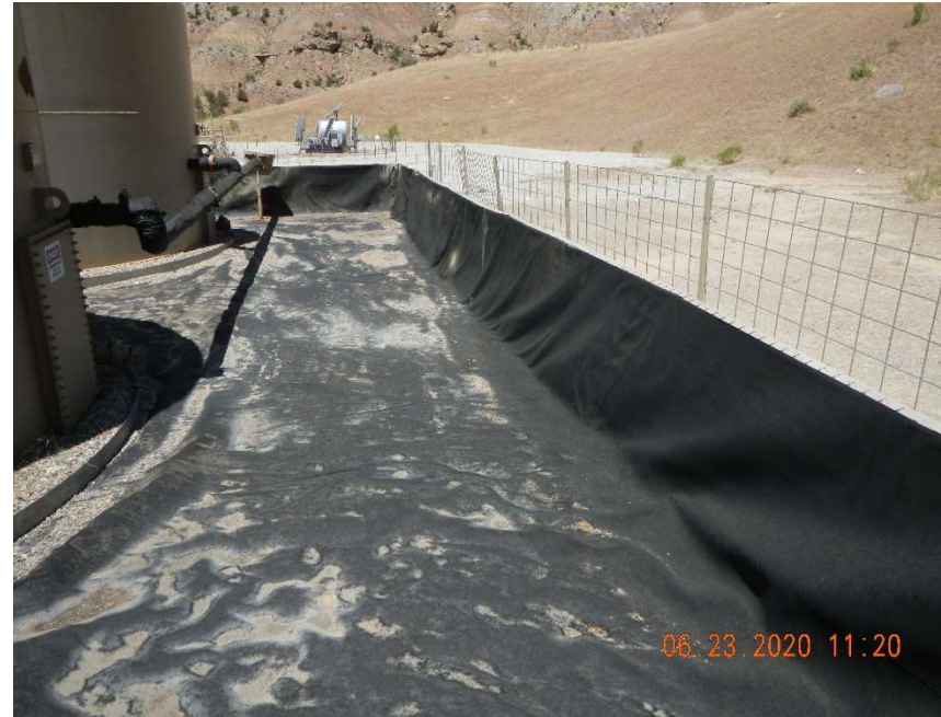
Tank battery secondary containment structure
