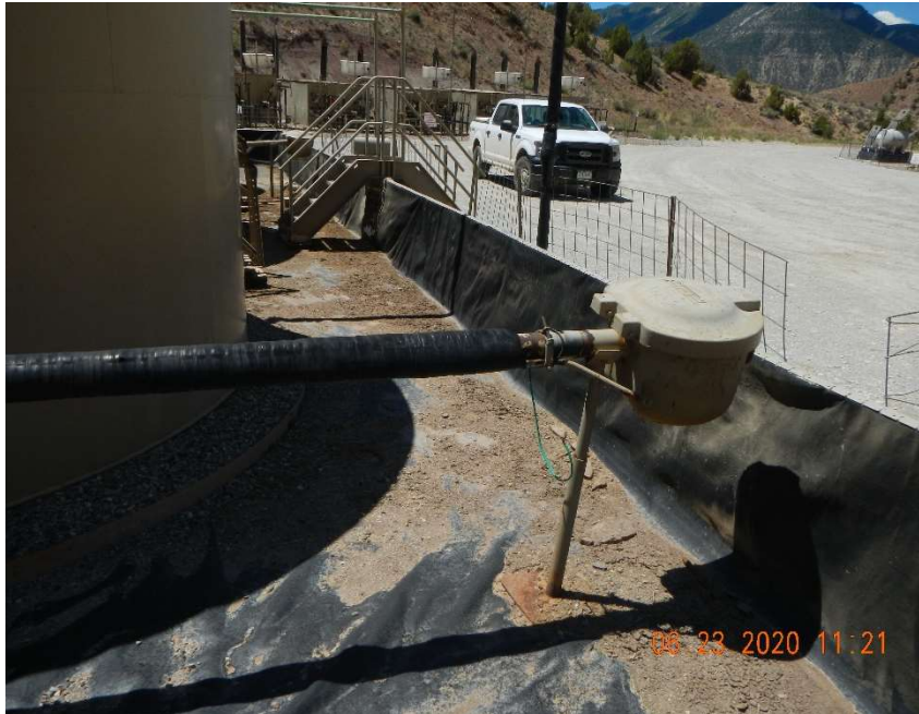
Tank battery secondary containment structure, note metal support directly on secondary containment liner
