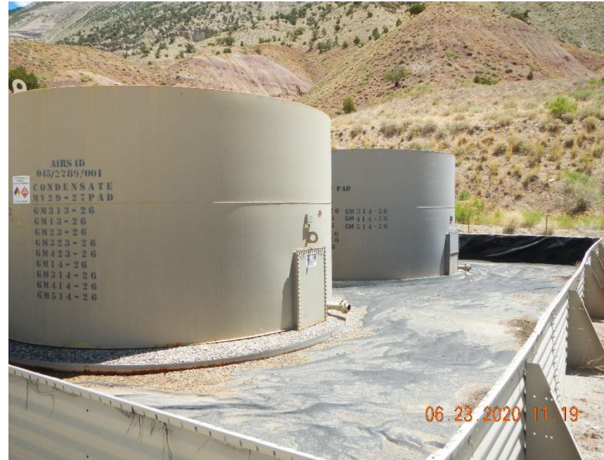
Tank battery secondary containment structure
