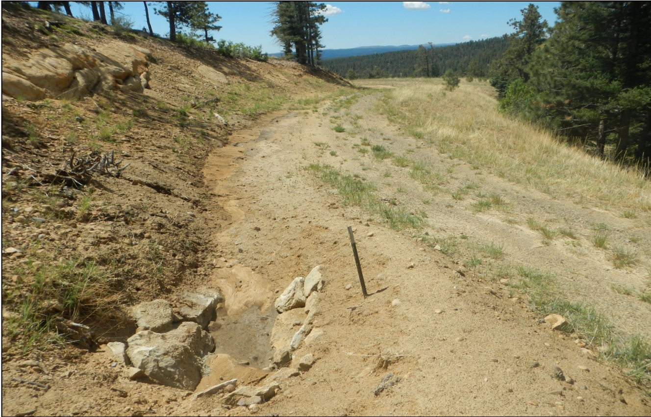
Photo 5. The culvert near the location has been cleaned out and maintained.
