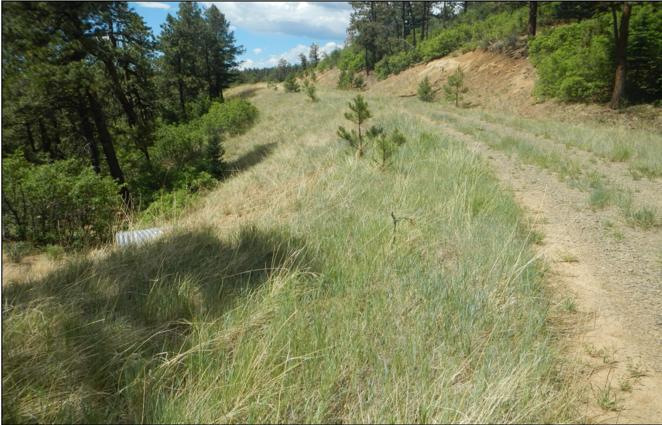
Photo 10. Facing back southwest along the access road. Vegetation is well established along the road.
