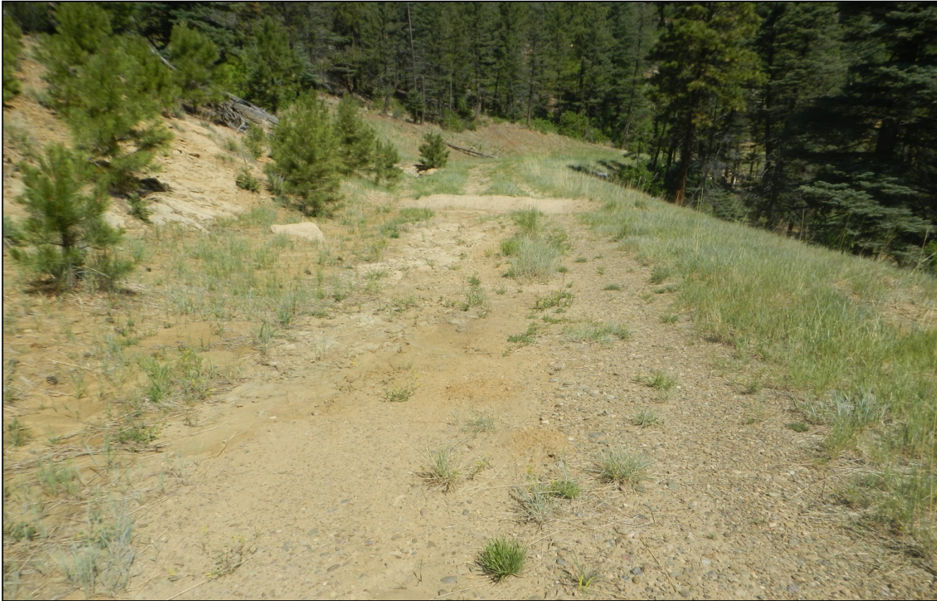
Photo 1. Facing northwest near the beginning of the access road. The road remains per approved variance request.
