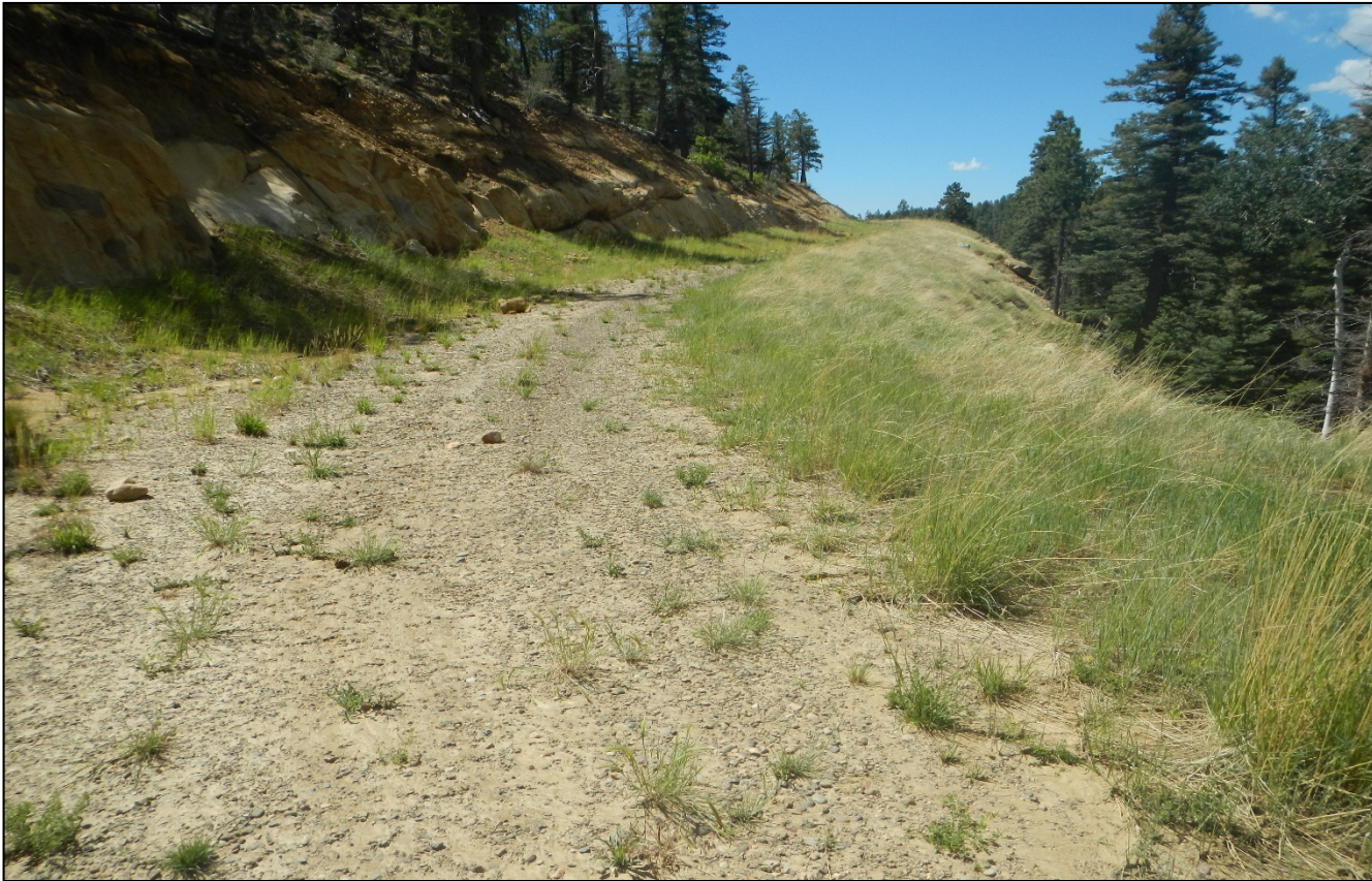
Photo 3. Further along the access road. The road is stabilized and maintained.
