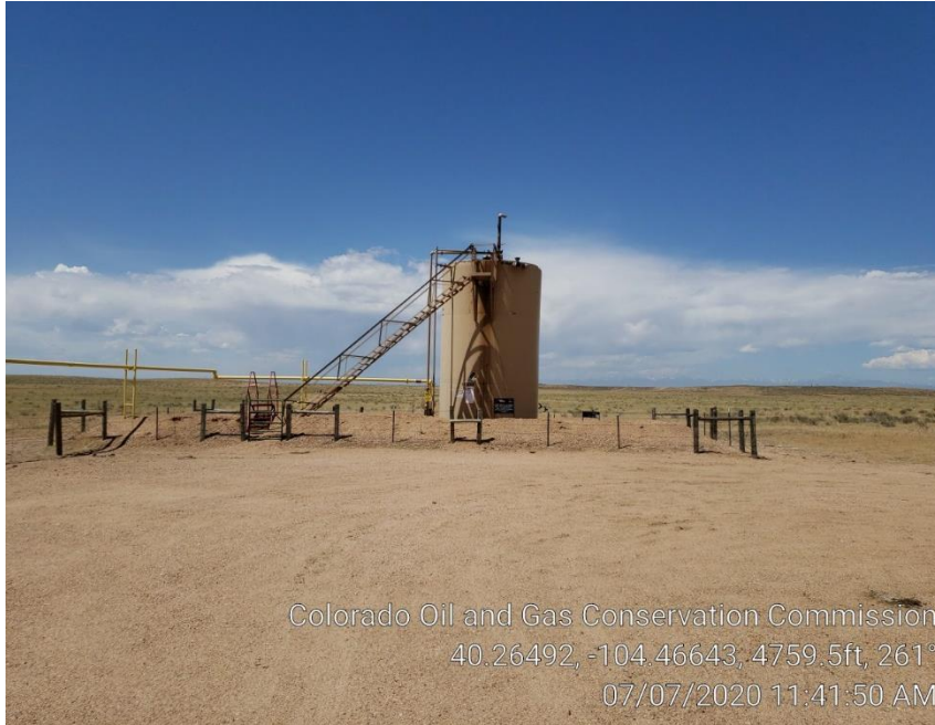
Photo #3 Tank Battery
